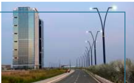
PU PAINTED BEND POLE
