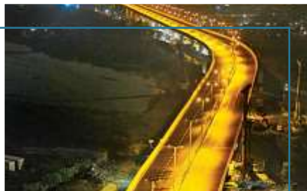
MUMBAI FREEWAY STEPDRAWN POLES
